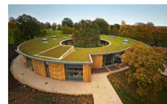
Figure 25. Example Green Roof
