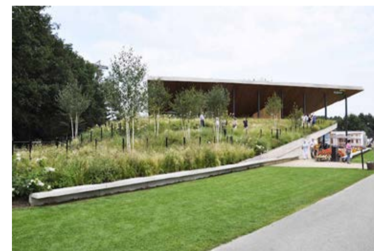
Figure 20. Example Green Roof
