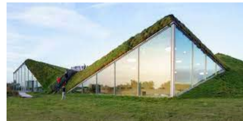
Figure 25. Example Green Roof
